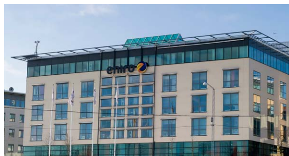
Solna Hilton 3. As at June, 29 Klöver signed an agreement of purchase of one property in Frösunda consisting of nearly 18,500 sq.m mainly office area, divided between three buildings. Klöver took possession of the property 5 July.
