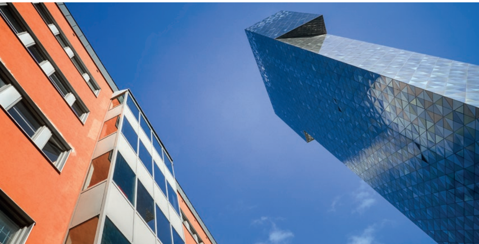
The property Helgafjäll 5, next to the Victoria Tower and Kistamässan, in central Kista.
