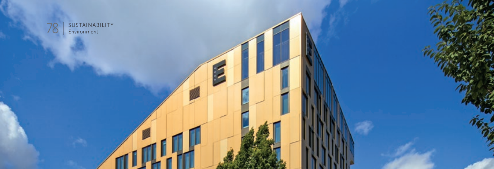
The property Kungsängen 10:2 which in 2017 was classified as Miljöbyggnad Gold.
