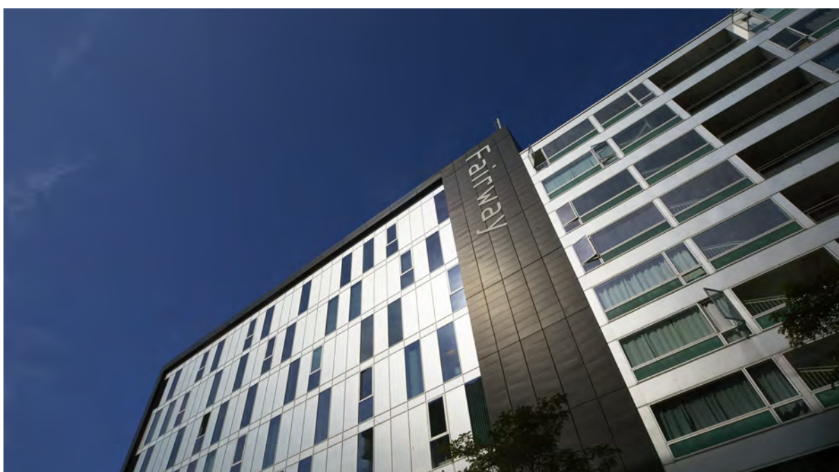
The property Fairway House in Copenhagen, one of the four properties in Denmark that Klöver, during the second quarter, signed contracts to acquire
