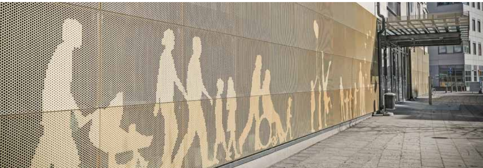
The property Hilton 3 in Solna has been totally refurbished and customized for the EU agency ECDC. Moving in took place during the first quarter of 2018.
