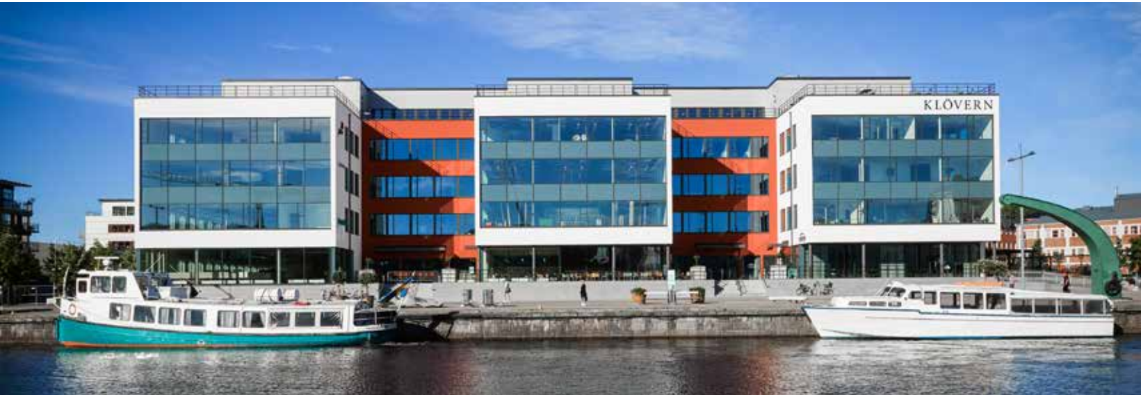
The property Pinassen 3, known as Skeppet, has been built directly by the water at Inre Hamn in Karlstad.
