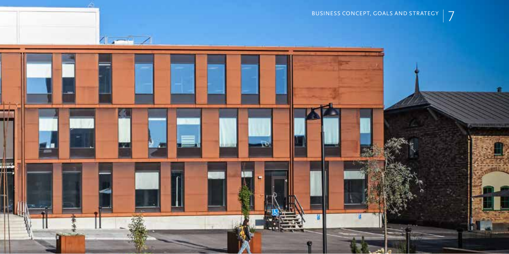
The property Gamlestaden 39:13 in Gothenburg.
